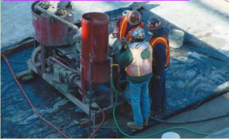
Mixing and pumping equipment
